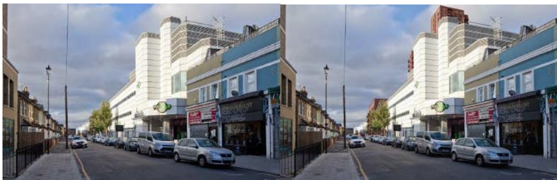
Figures 42 and 43: view from Frith Road, facing north west towards the Site without (left) and with (right) proposal
