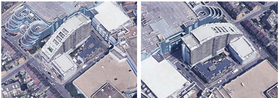
Figures 4 and 5: birds eye views of the existing building
