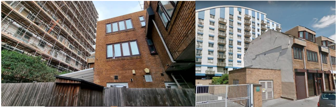
Figures 62 and 63: relationship between existing building and Keeley House close up (left) and at a distance (right)
